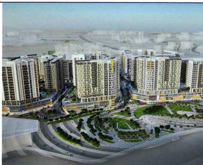
HLG Contracting will construct Expo Village, five 16-storey residential towers in Dubai
